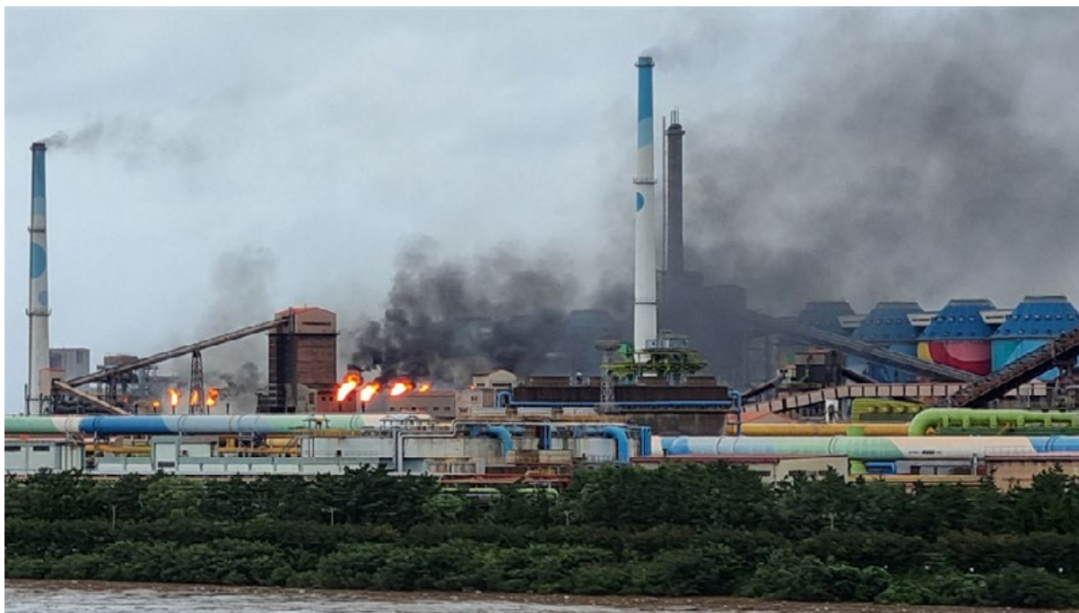
Figure 21: Fire at Posco's Pohang steel plant caused by Typhoon Hinnamnor ( The Korea Times, 2022 )
