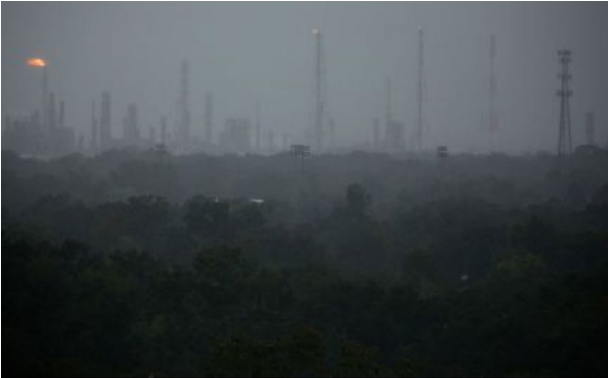
Figure 12: A Royal Dutch Shell refinery as Hurricane Ida made landfall ( CNN, 2021 )
